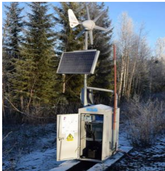
Figure 7. An example of wayside lubrication system integrated with micro-scale solar panels and wind turbines [14]
