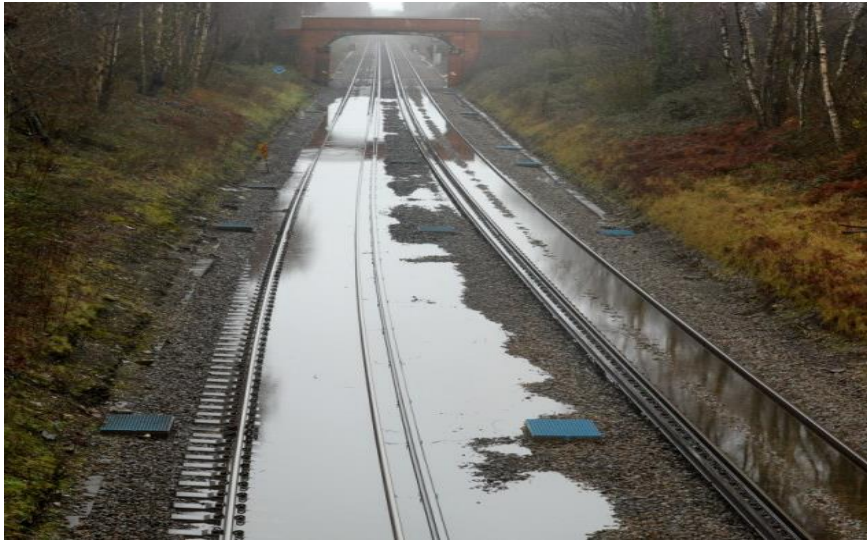
Figure 15. An example from England how the excessive rainfall damages on track and its surroundings [51]
