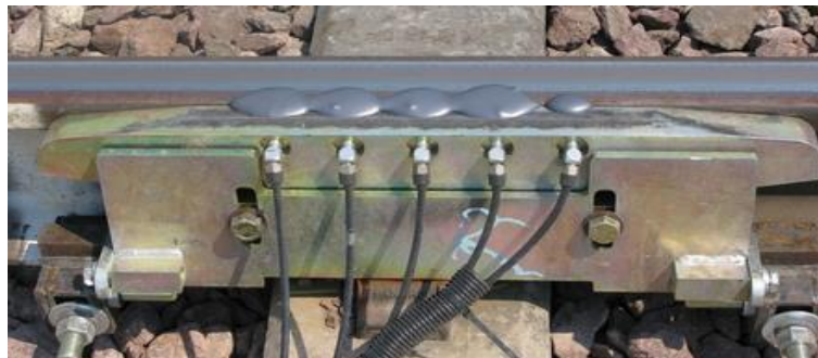
Figure 5. An example of the wayside lubrication system for Top-on Rail (ToR)[10]
