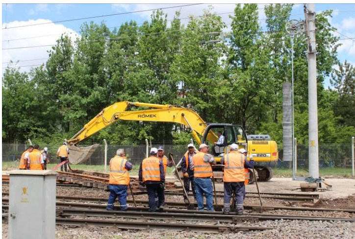
Figure 2.7 - Illustration of old S&C section being removed.
