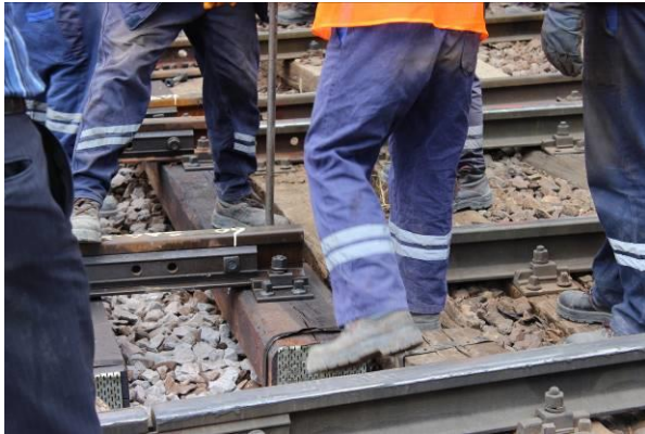
Figure 2.9 - Installation of insulated block joints
