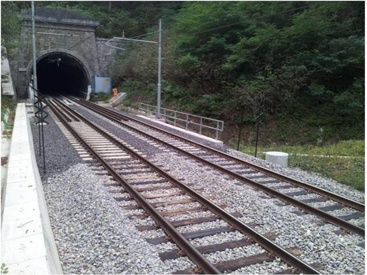
Figure 66: Transition zone – final state after rehabilitation
