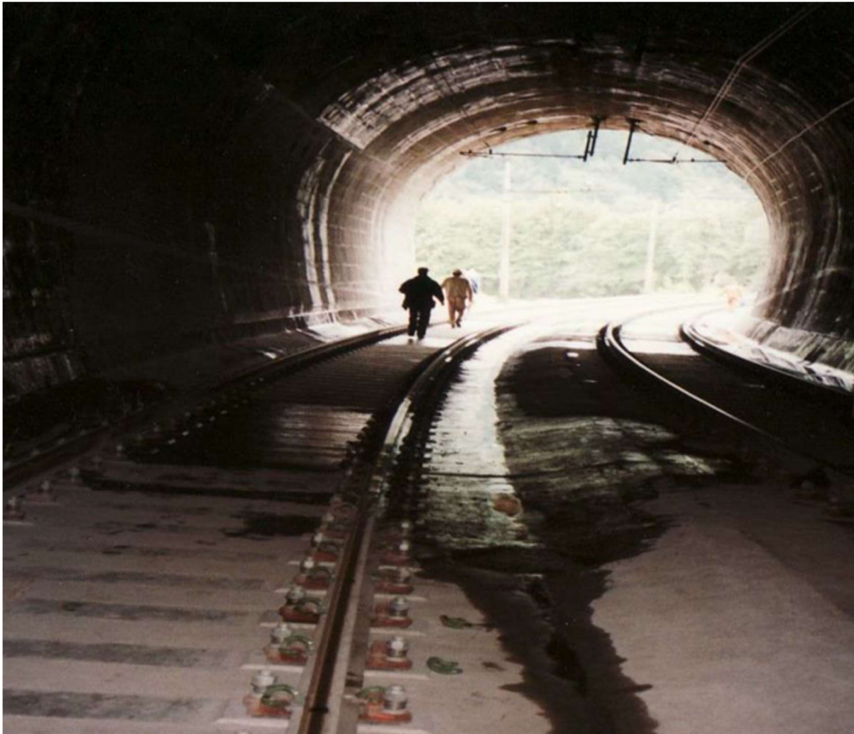
Figure 63: Tunnel Poganeč after rehabilitation
