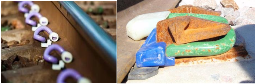
Figure 3 – Pandrol e-Plus and Fast clip (Trafikverket 2015a)
