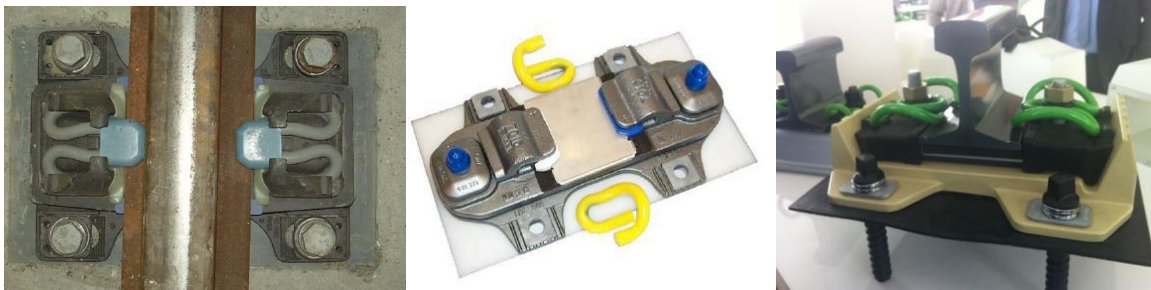
Figure 4 – Pandrol VIPA S, Pandrol VIPA F1 and Vossloh DFF (Trafikverket 2015a)
