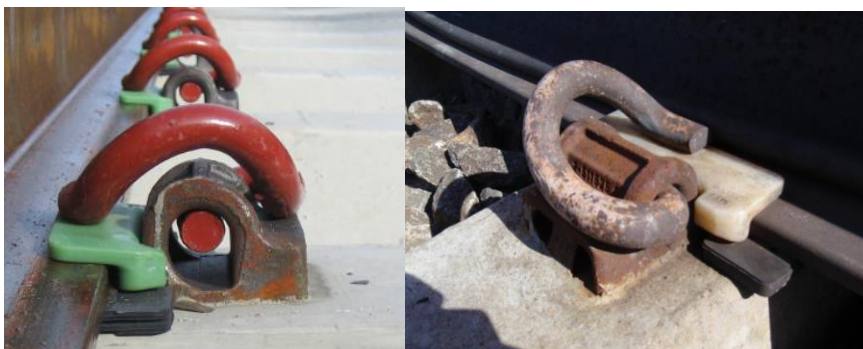
Figure 2 – Pandrol E-clip (1817) and Deep-Post (Trafikverket 2015a)
