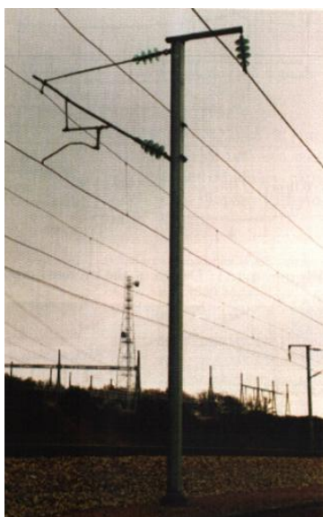
Figure 4.20 - Pole with pull-off contact wire support as adopted on the Paris-Strasbourg line
