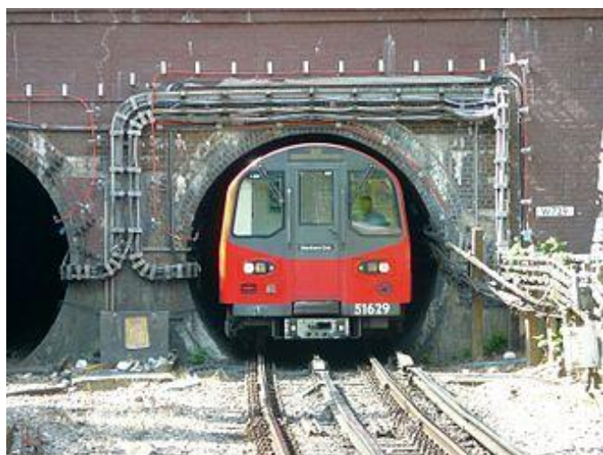
Figure 3.22 – Fourth rail and third rail 11
