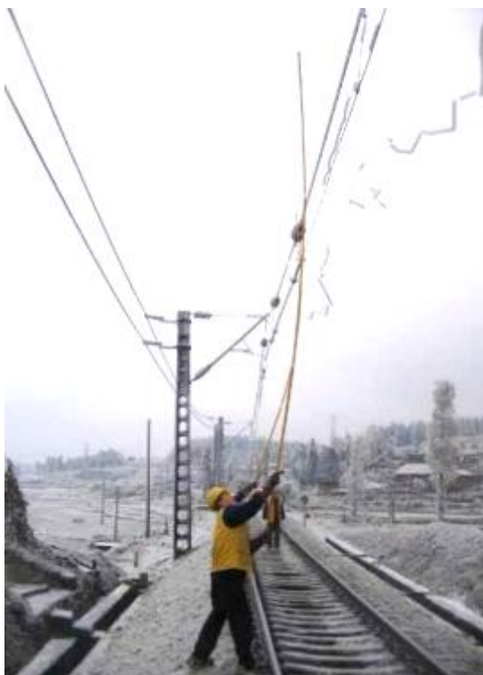
Figure 4.26 – Manual de-icing from ground (26)
