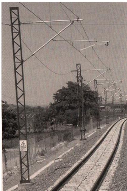
Figure 4.17 - Cantilever of the La Sagra-Toledo line
