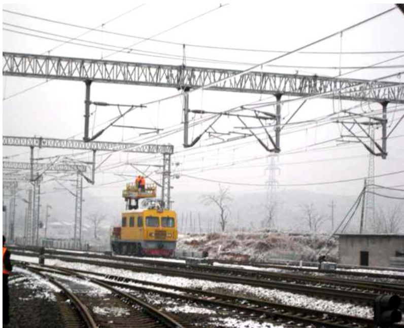
Figure 4.25 – Manual de-icing from a mobile platform (26)
