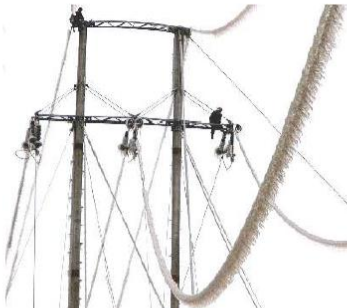
Figure 4.28 – Icing of high-voltage line (26)
