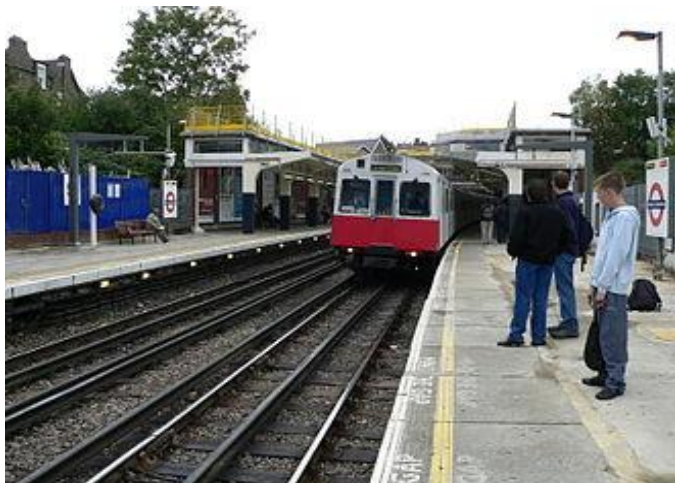
Figure 3.23 – Rail station in London with third rail and fourth rail
