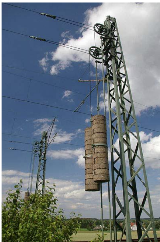
Figure 3.12 – Example of tensioning line 6
