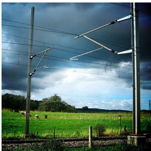
Figure 4.13 - Overhead lines on contact line design BN 160 12
