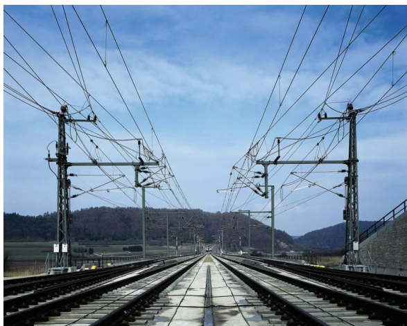
Figure 3.3 – Catenary and Railway Power Supply 5
