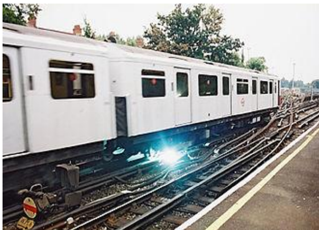
Figure 3.18 – Arc which appear in third rail systems
