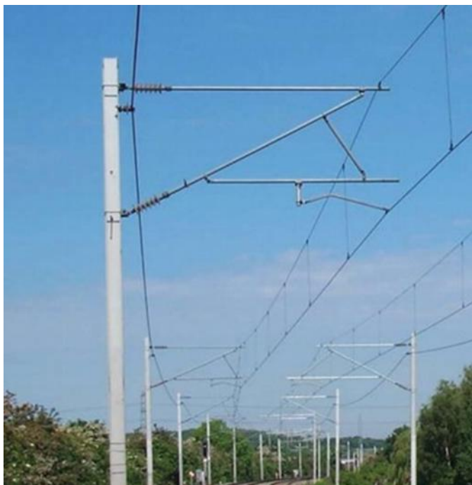
Figure 4.34 – Simple catenary equipment 14
