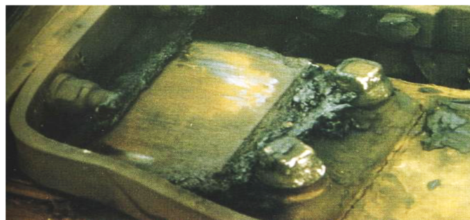
Figure 3.1 - Dry slide baseplate (Hassankiadeh, 2011)
