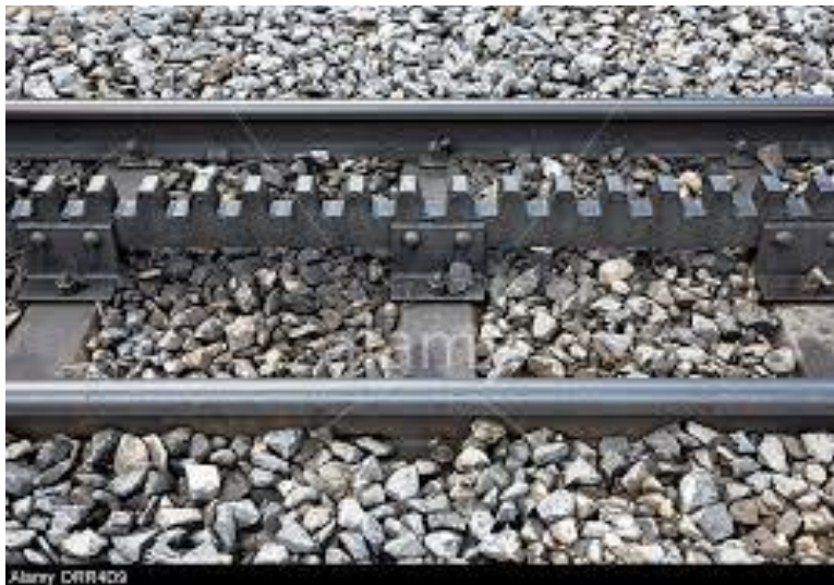
Figure 2.2 - Rack Railway detail 24
