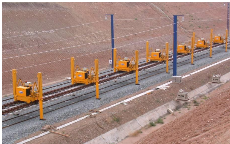
Figure 2.14 - Installation of a switch panel by portal cranes. (source: COMSA).
