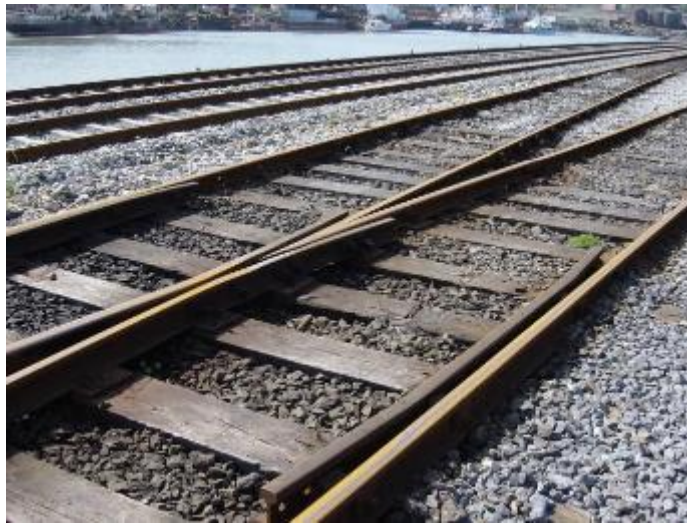
Figure 1.4 – Wooden sleepers track 3
