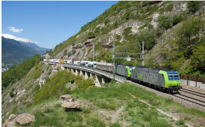
Figure 1.2 - Cutting formation of Lötschberg - Bahn, Switzerland 2
