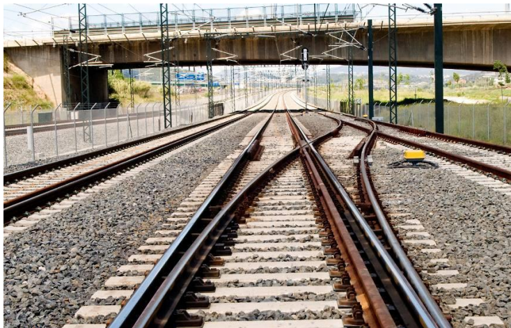
Figure 2.9 - Switch in a dual gauge line in Spain (source: Adif)
