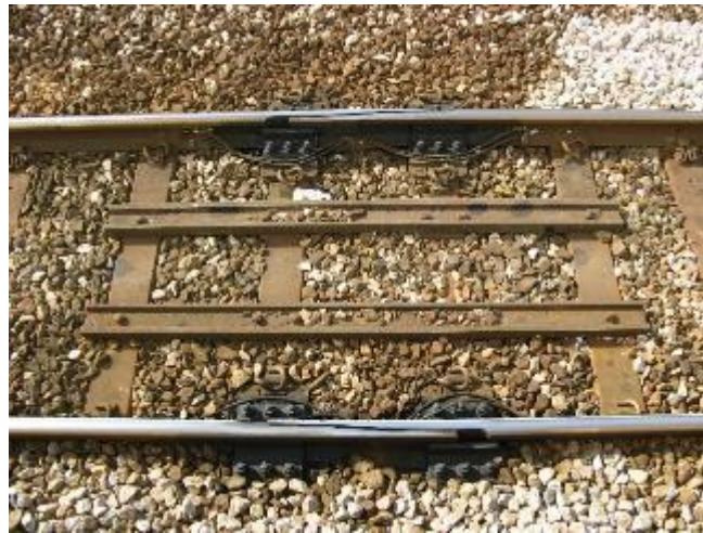
Figure 1.31 - An expansion joint on the Cornish Main Line, England
