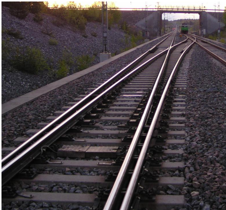
Figure 2.6 - UIC60-760-1:15 turnout in Härad. (17)
