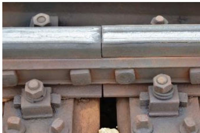
Figure 1.21 - Rail Joints Example at RCCF partner
