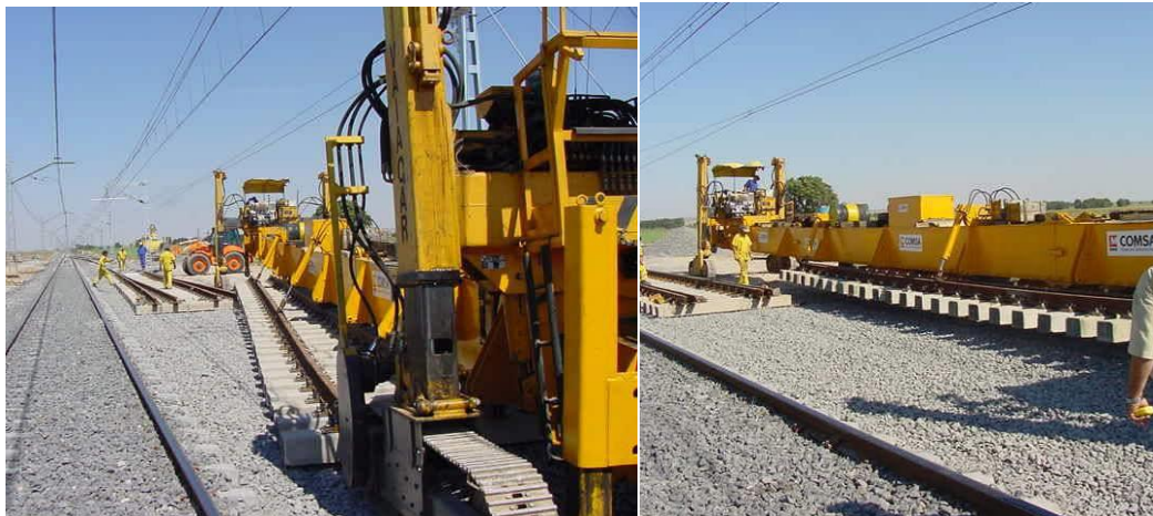
Figure 2.13 - Installation of a switch with VAIACAR crane-beam system. COMSA.
