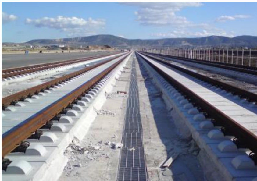
Figure 2.23 - Ballastless Track / Slab Track system 32
