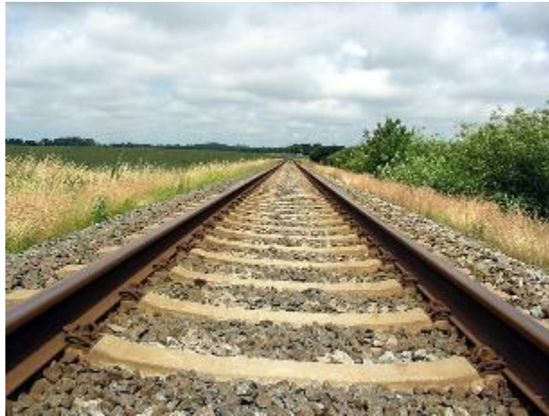
Figure 1.6 - Concrete sleepers 5
