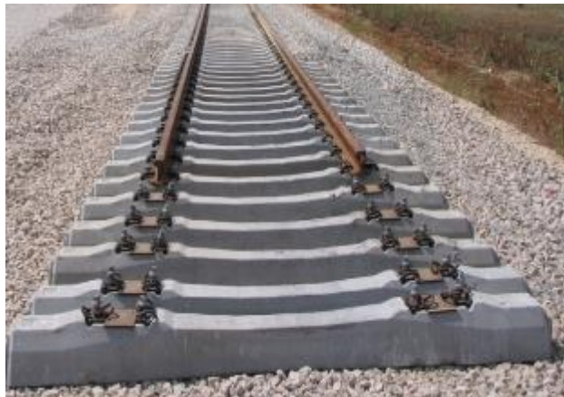
Figure 1.7 –Installing concrete sleepers
