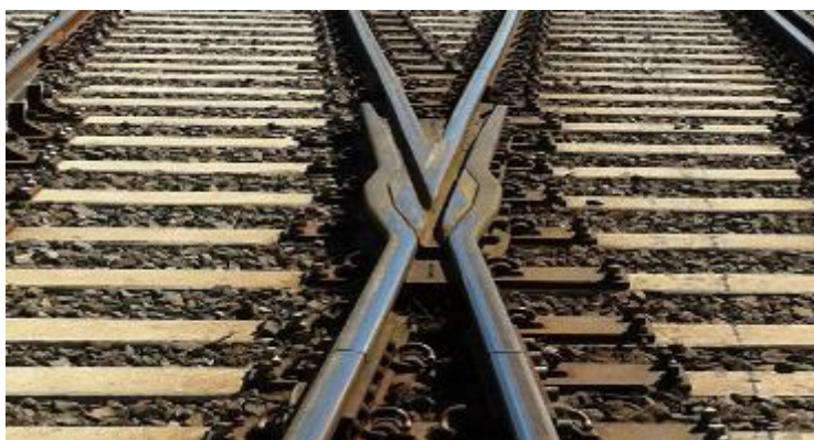
Figure 1.39 – Example of Crossings
