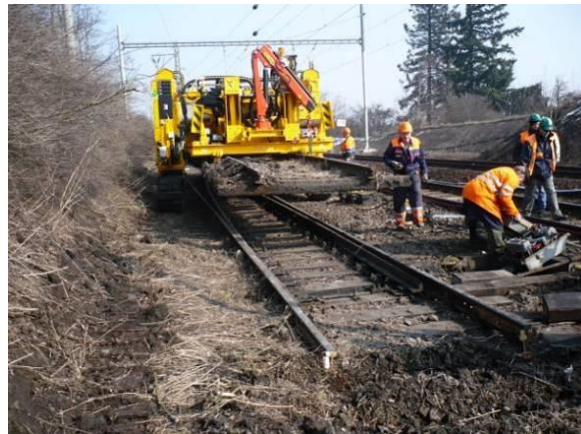
Figure 2.16 - Replacement of a switch using Desec system (source: Skanska).
