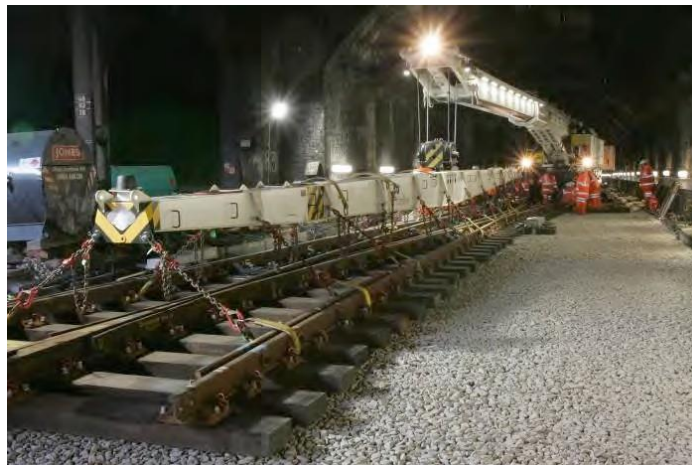
Figure 2.15 - Installation of a switch using the Kirow crane (source: Balfour Beatty).
