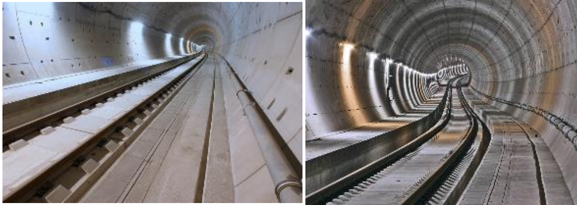
Figure 2.22 – Tunnelling Ballastless Track / Slab Track 31
