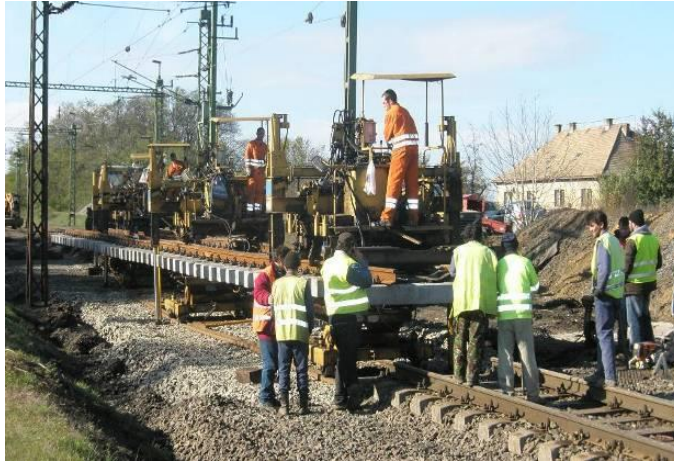
Figure 2.17 - Replacement of a switch using Geismar UWG system (source MAV)
