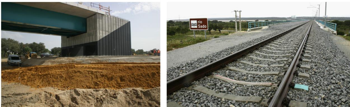
Figure 14 Side view of the transition zone before construction and general view of the track [4]
