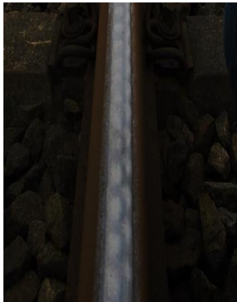
Figure 2-5. A location with corrugation recorded on Dutch railway network
