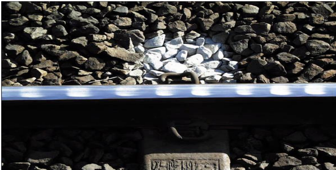
Figure 5.1: Short pitch corrugation
