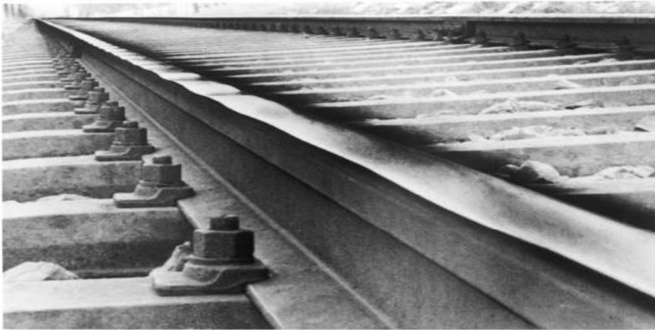
Figure 5.2: Long pitch corrugation
